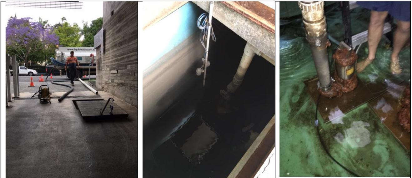
**Lees Liquid waste sucking out the balance of the water and sludge from the tank. Note access via a VERY heavy cement hatch in the driveway which had not been opened in 12 years. The empty tank with sludge. Clean tank and 10cm of new rainwater. Both pumps had been knocked off the pipes and were lying on the floor of the tank. Now reconnected and serviced, and the inlet flow redirected so it doesn't directly hit the pumps.**
